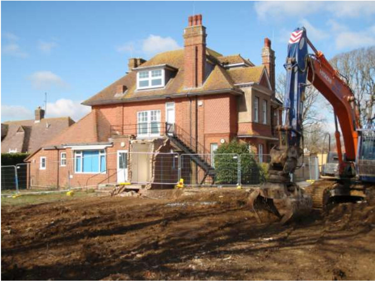
Plate 3. The site showing ground strip of topsoil, facing north-west
