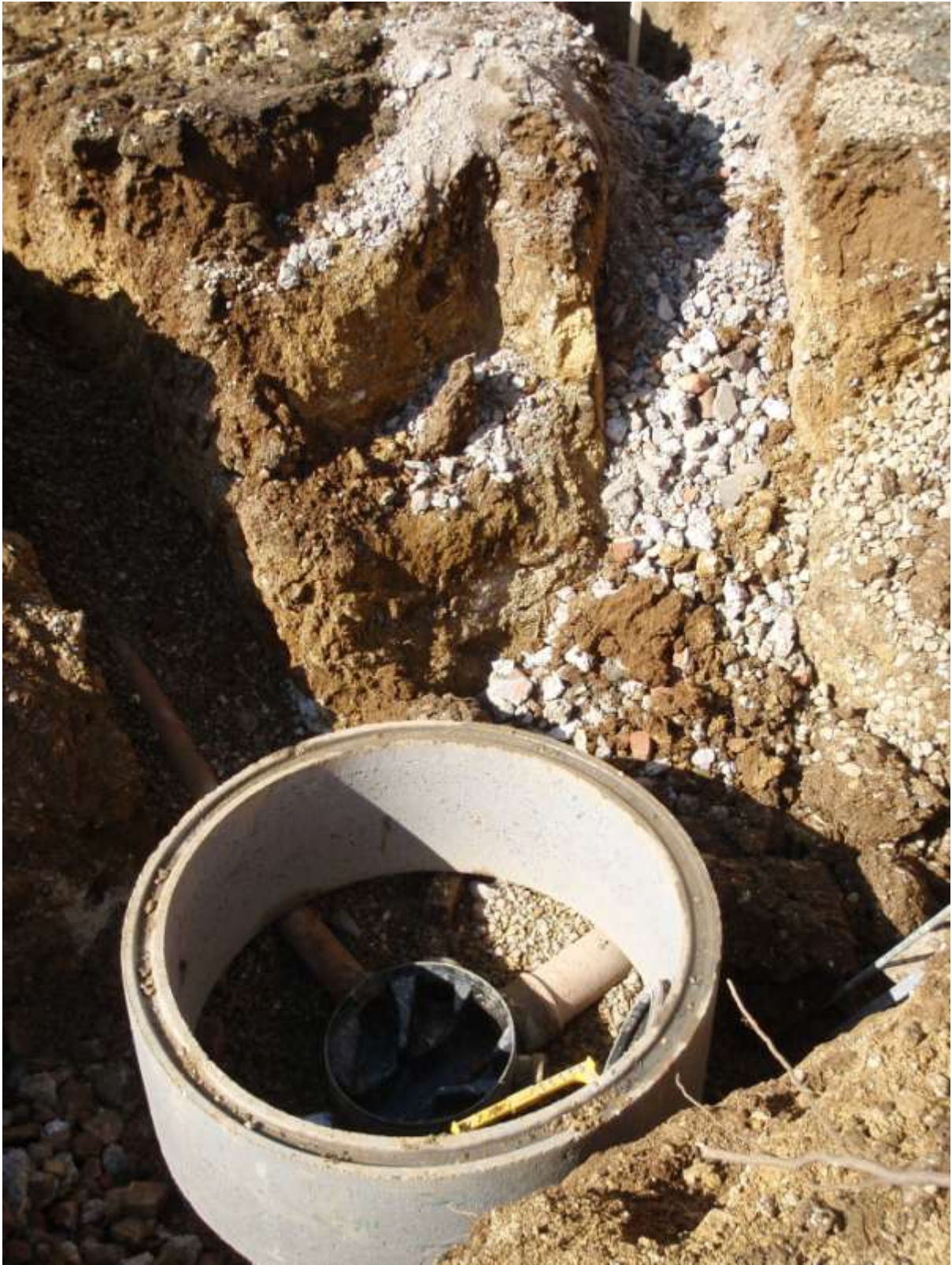
Plate 6. Excavation of drainage runs
