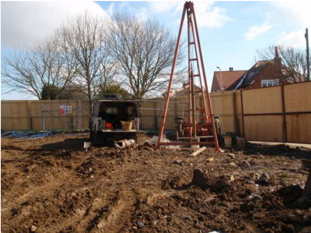
Plate 2. General view of site with piling in process, facing east
