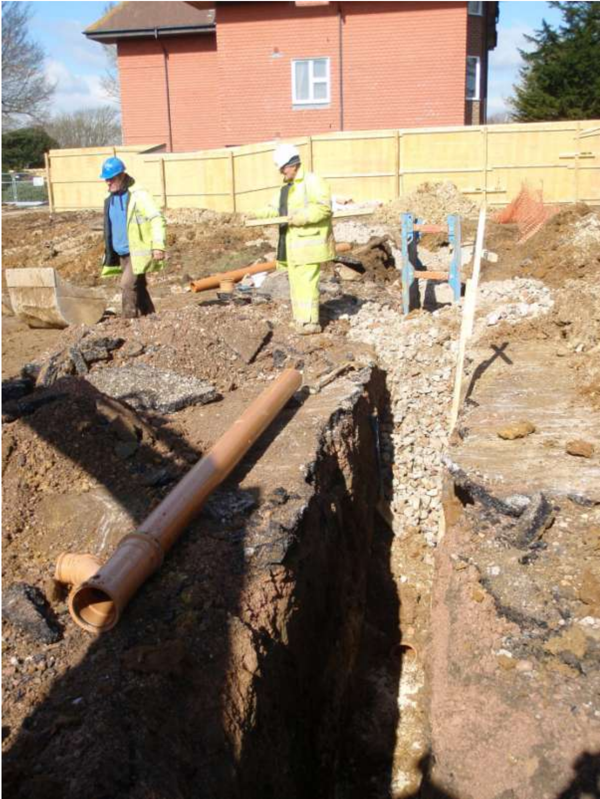
Plate 5. Excavation of drainage runs
